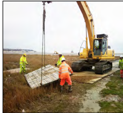
Positioning of Timber Mats
